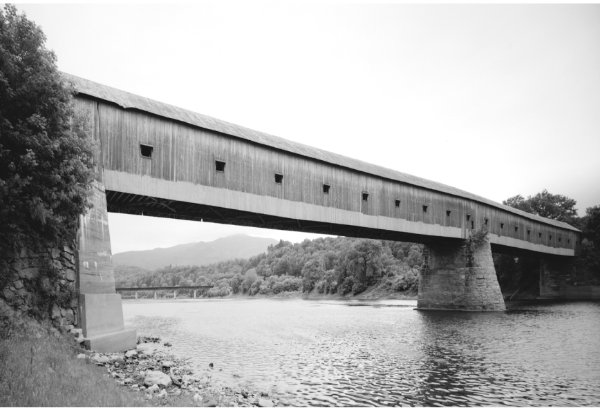
The Cornish-Windsor covered bridge (1866) spanning the Connecticut River, between Cornish, N.H., and Windsor, Vt., 1984
